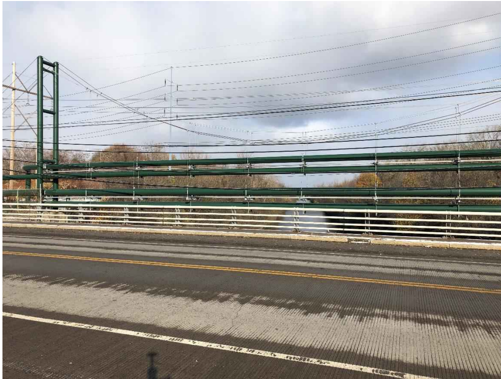
Figure 4-3.13 Simulation of Proposed Line on Existing ROW looking north from canal crossing of Buffalo Road
