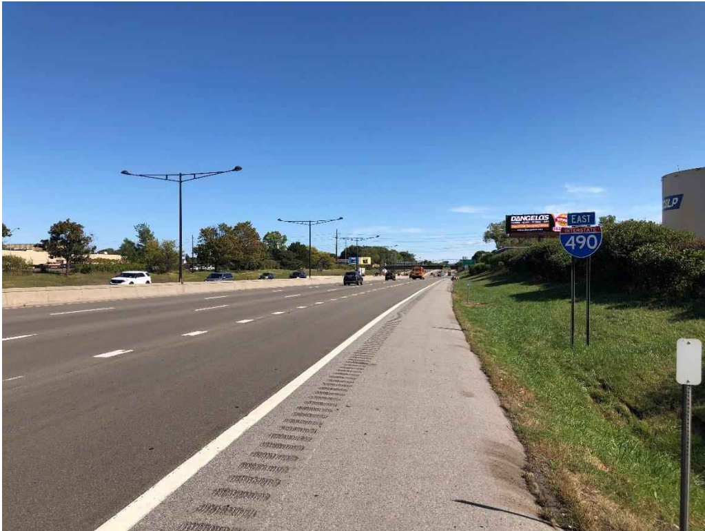
Figure 4-3.14 Existing ROW looking east from shoulder of 490 (east), taken October 8, 2019
